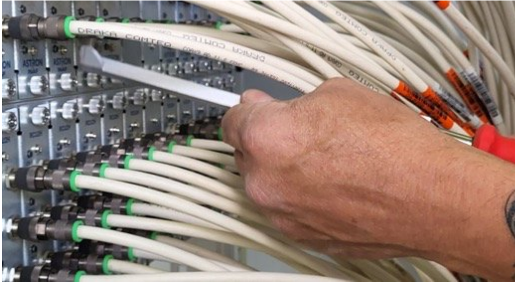
Dismantling a LOFAR1 station ©ASTRON
